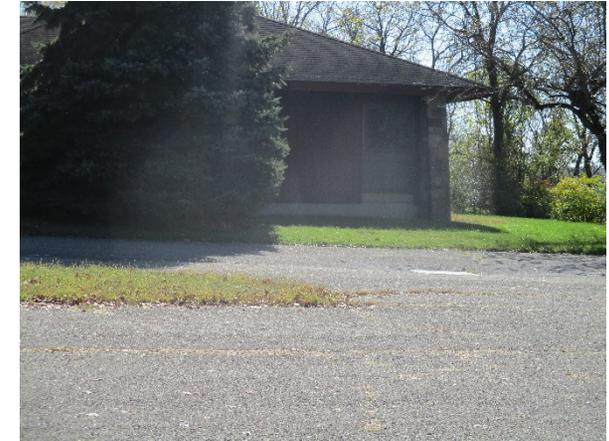
The southernmost parking spaces in the parking lot can be converted to pervious pavement to capture and infiltrate stormwater runoff from the parking lot. Downspout planter boxes can be constructed along the building to allow roof runoff to be captured and treated. A preliminary soil assessment suggests that more soil testing would be required before determining the soil's suitability for green infrastructure.
