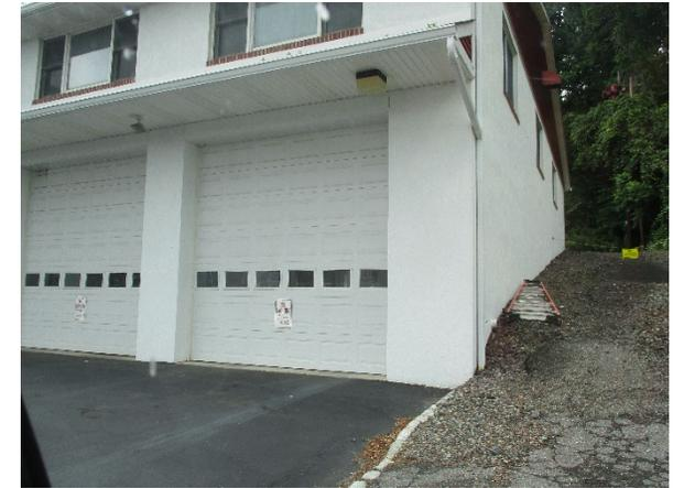
A cistern can be installed at the southeast downspout of the building to harvest rainwater from the roof. Captured rainwater can be used for non-potable uses such as washing vehicles. A preliminary soil assessment suggests that the soils have suitable drainage characteristics for green infrastructure.
