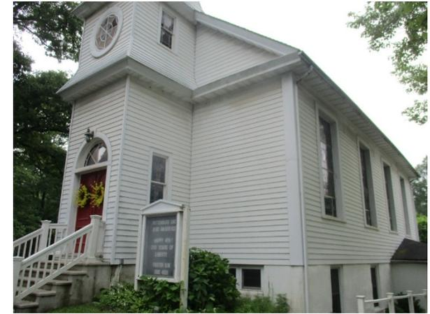
A rain garden can be installed at the east side of the building to capture, treat, and infiltrate stormwater runoff from the rooftop via the connected downspout. A preliminary soil assessment suggests that the soils have suitable drainage characteristics for green infrastructure.
