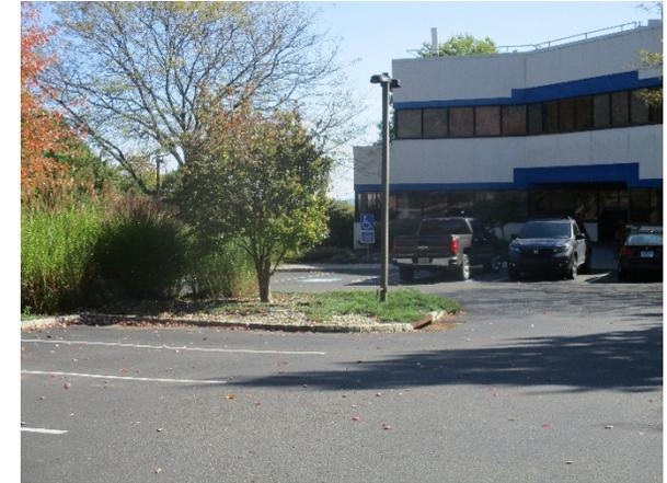
Parking spaces west of the building can be converted to pervious pavement to capture and infiltrate stormwater runoff from the road and parking lot. A preliminary soil assessment suggests that more soil testing would be required before determining the soil's suitability for green infrastructure.
